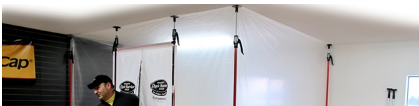
Temporary plastic sheeting system with telescopic supports
